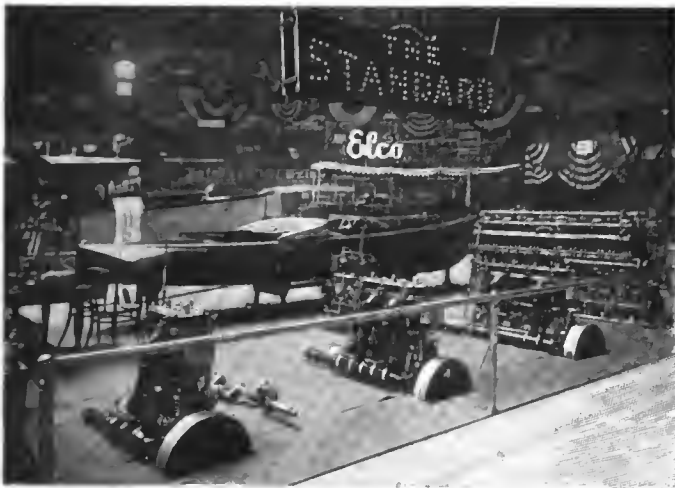
LARGEST ENGINE TO THE RIGHT IS 300-HORSEPOWER. Exhibited by Standard Motor Construction Company, Jersey City, N. J.
